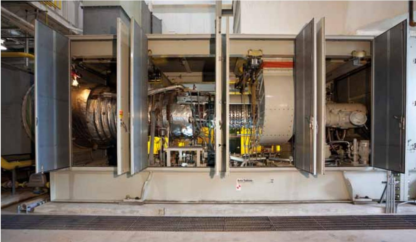
**Figure 25:** A Solar Turbines Titan 130 generator set provides district heating and electricity to London District Energy in London, Ontario, Canada.
