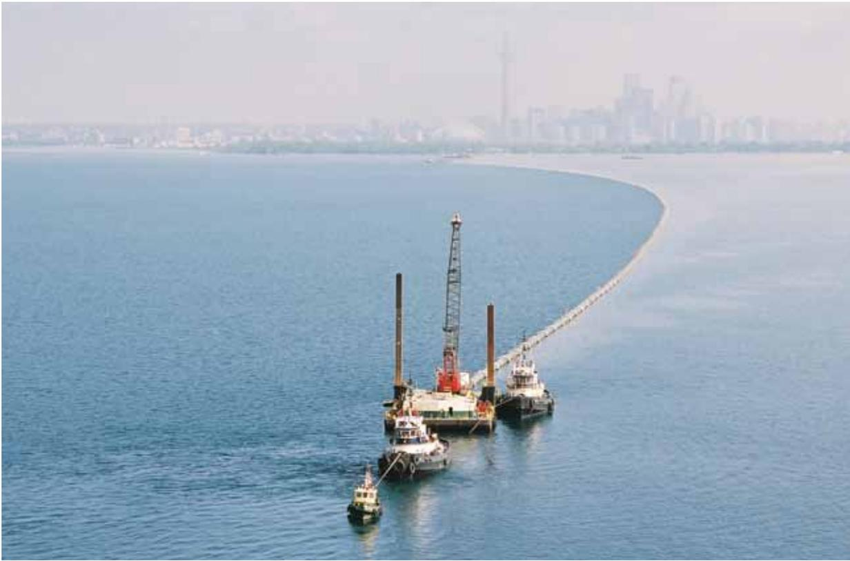
**Figure 12:** Enwave's Deep Lake Water Cooling uses the icy water of Lake Ontario to provide renewable cooling for the city of Toronto.
