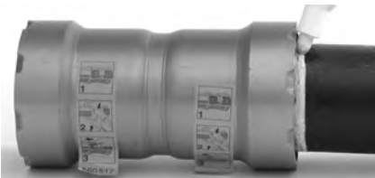
Figure 7 – Marking the Pipe After Fully Inserting Pipe
