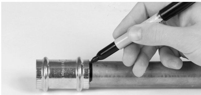
Figure 8 – Marking the Tubing After Fully Inserting Tube
