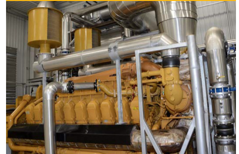
Toromont Power Systems installed two high-efficiency Cat® G3520C natural gas generator sets providing 4 MW of power to anchor the CHP system.
