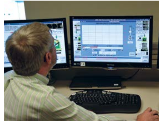
Network operations center
