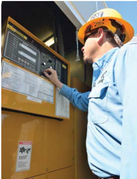
(L) A Cat G3520C genset backs up Orangeburg’s wastewater treatment plant. (R) Monthly load test.
