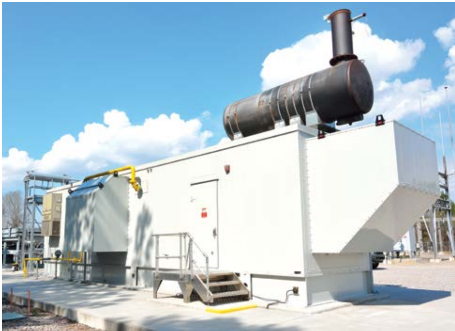
(L) A Cat G3520C genset backs up Orangeburg’s wastewater treatment plant. (R) Monthly load test.
