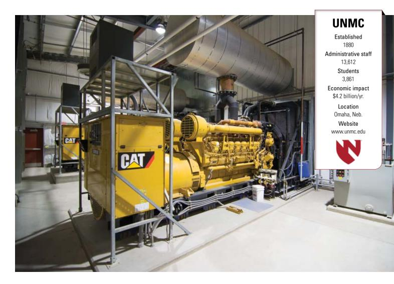
the operation of the generator sets and distribution circuit breakers. In the event of a power failure, a series of automatic transfer switches transfer the utility load to the generators, and maximum load is achieved within 10 seconds.
