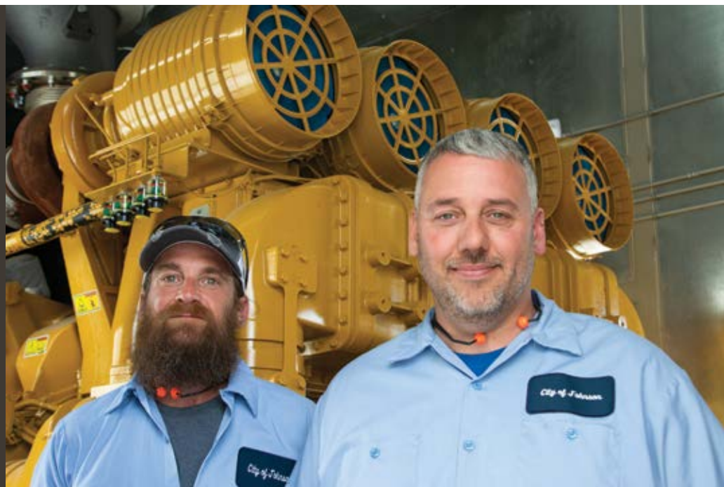
David Rohrenback, power plant superintendent (left) and Tyce McMillan, public works superintendent
